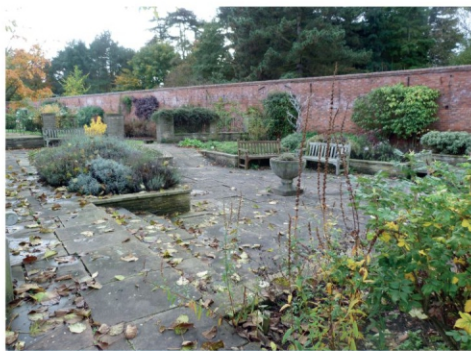
Wall of Kitchen garden Showing greenhouse roof supports.
