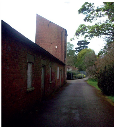
Header Tank, Elvaston Estate.
